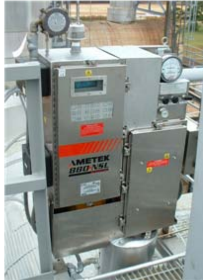
Fig 4a. Typical Analyzer Installation “Top of Pipe” Type Analyzer
