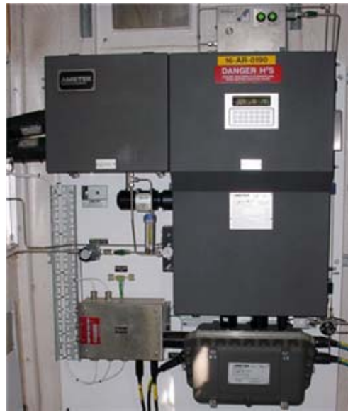
Fig. 4b. Typical Analyzer Installation “Sample Line Type” Analyzer
