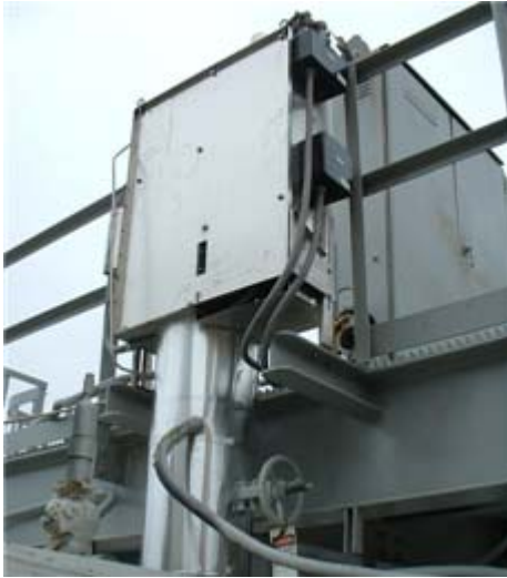
Fig 4a. Typical Analyzer Installation “Top of Pipe” Type Analyzer
