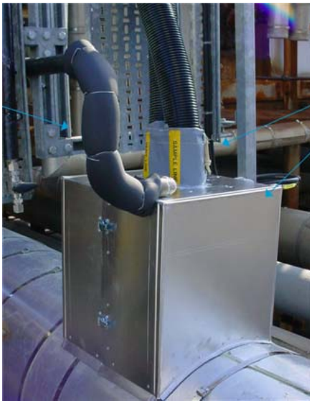
Fig. 4b. Typical Analyzer Installation “Sample Line Type” Analyzer
